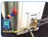
Vacuum with VG64-LX digital gauge
